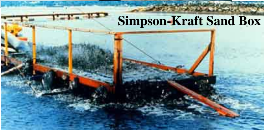
Sprayed slurry system placing sand at Soda Lake, WY
