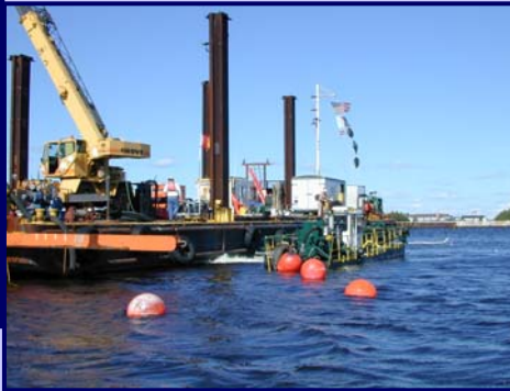
Manistique - Diver operated suction using dredge pumps
