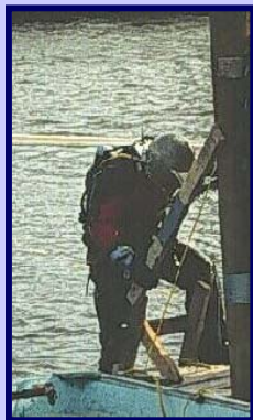
Manistique - Diver operated suction using dredge pumps
