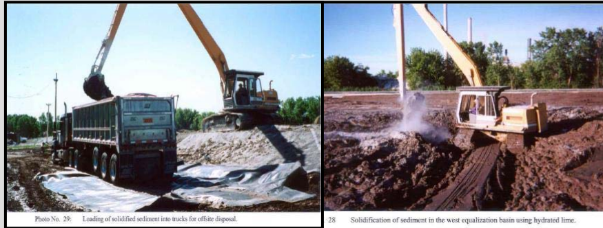
Photo No. 29: Loading of solidified sediment into trucks for offsite disposal.
