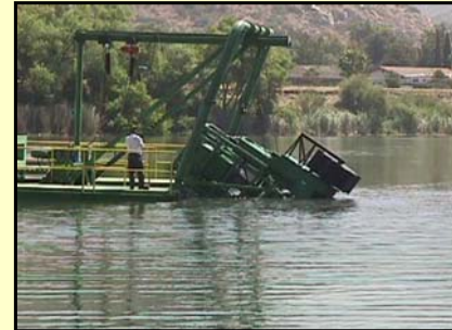
Eddy Pump on Tornado I
