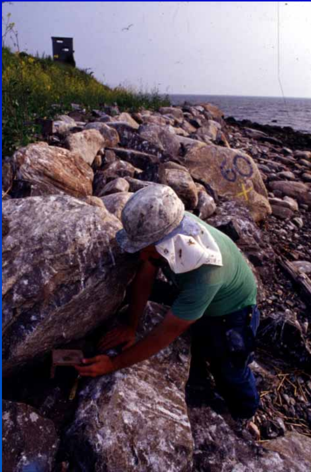
Adding chick shelter to secondary revetment on SW Shelf
