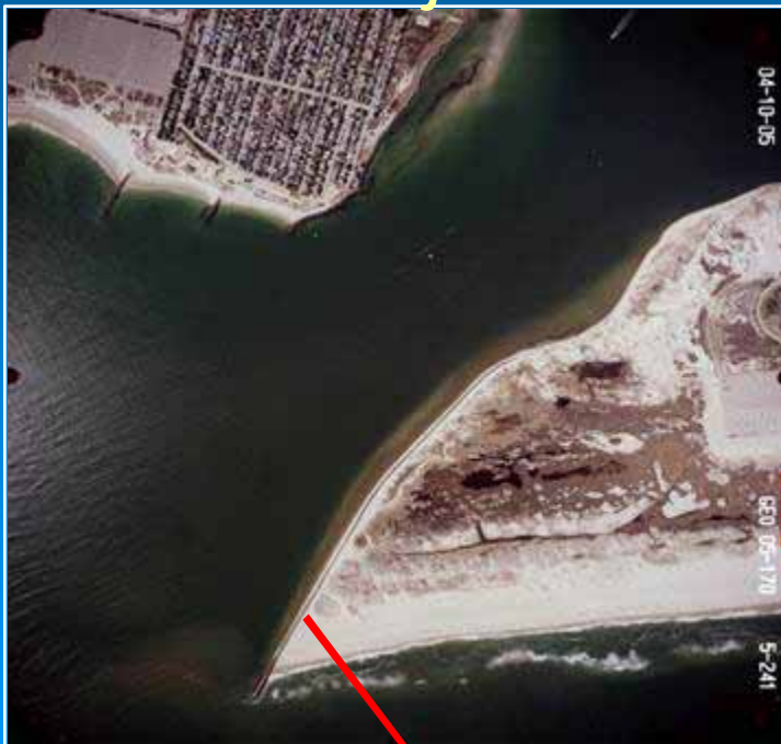
Jones Inlet Navigation Project
