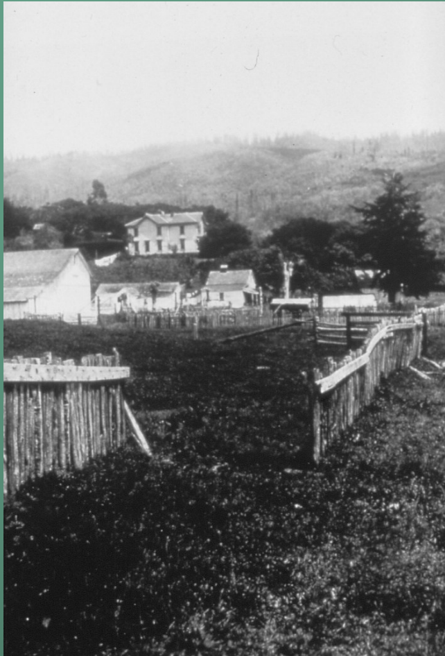
8.5 feet offset in San Andreas fault from 1906 earthquake. Marin County
