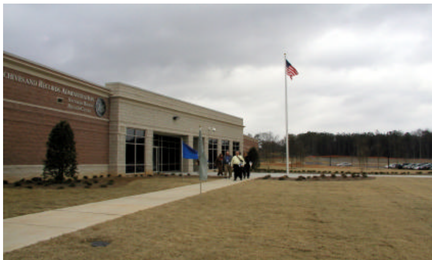
Federal Records Center, Ellenwood, GA, January, 2005
