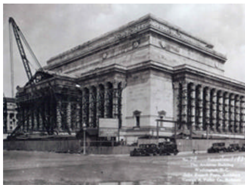
The construction of the National Archives Building, June 1934.
