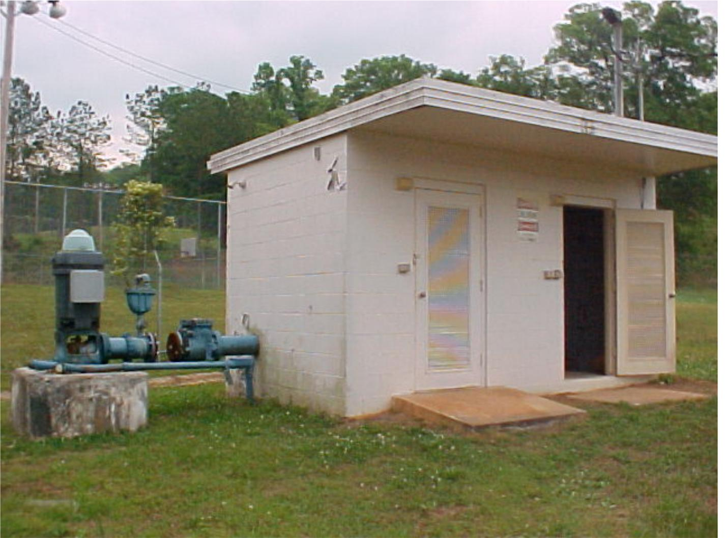
Figure 1: Grant Street Well – Note missing section of pipe.
