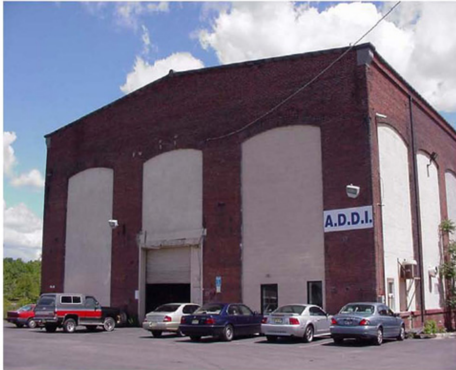
Photograph 1. Former Zonolite/W.R.Grace building, Hamilton Township, Mercer County, New Jersey.
