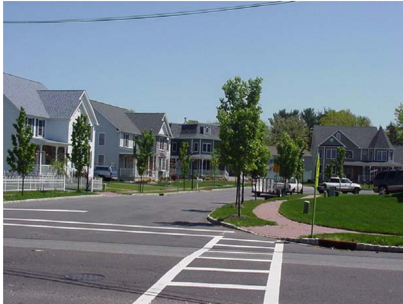
Photograph 1: Residences built on Mercer Rubber Company site
