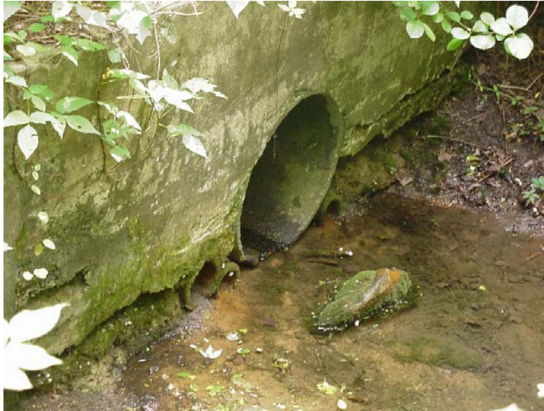
Photograph 5: Outfall pipes draining into the unnamed creek
