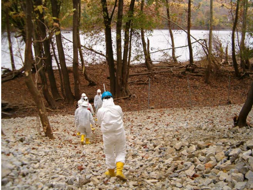
Photograph 3: Riprap on the western portion of the Crown Vantage Landfill site, October 26, 2004
