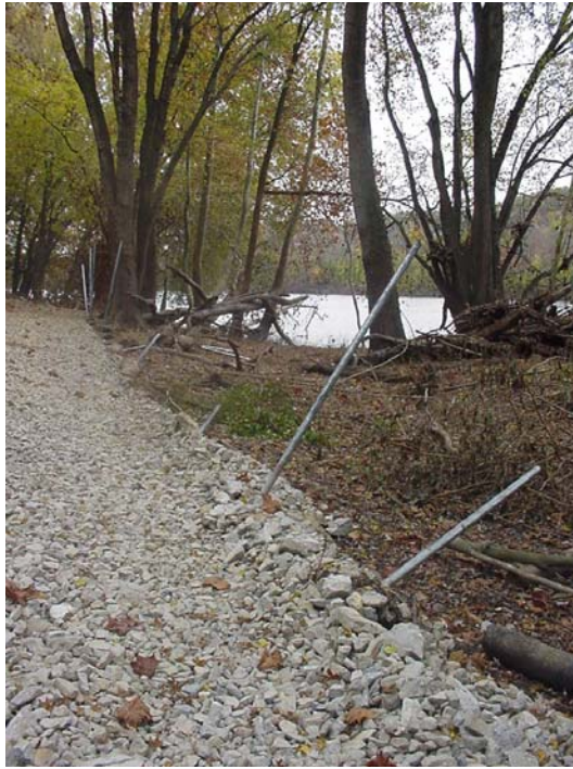
Photograph 5: View of fallen fence posts on the western portion of the Crown Vantage Landfill site, August 11, 2005
