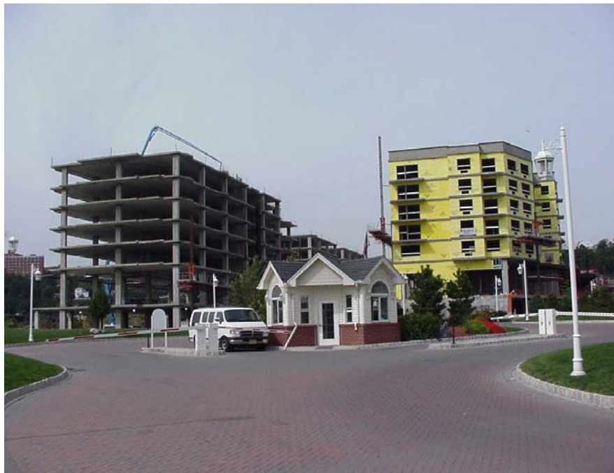
Photograph 4. The guard house situated on the landfill
