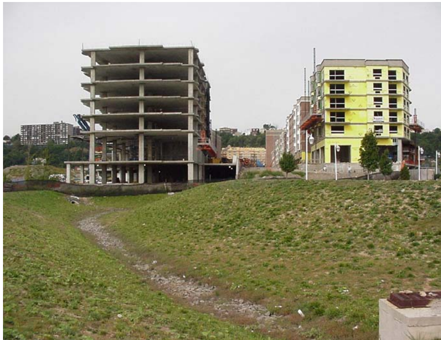
Photograph 2. The detention basin at the Celotex Corporation site
