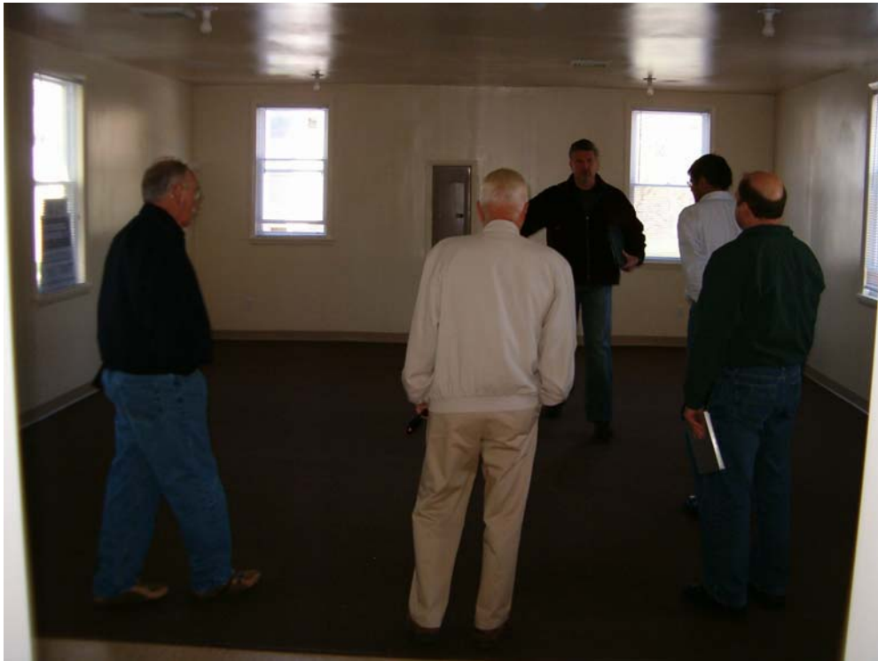
Building interior of former Rooms 2 & 3 where Adrow Chemical Company conducted mercury refining operations.
