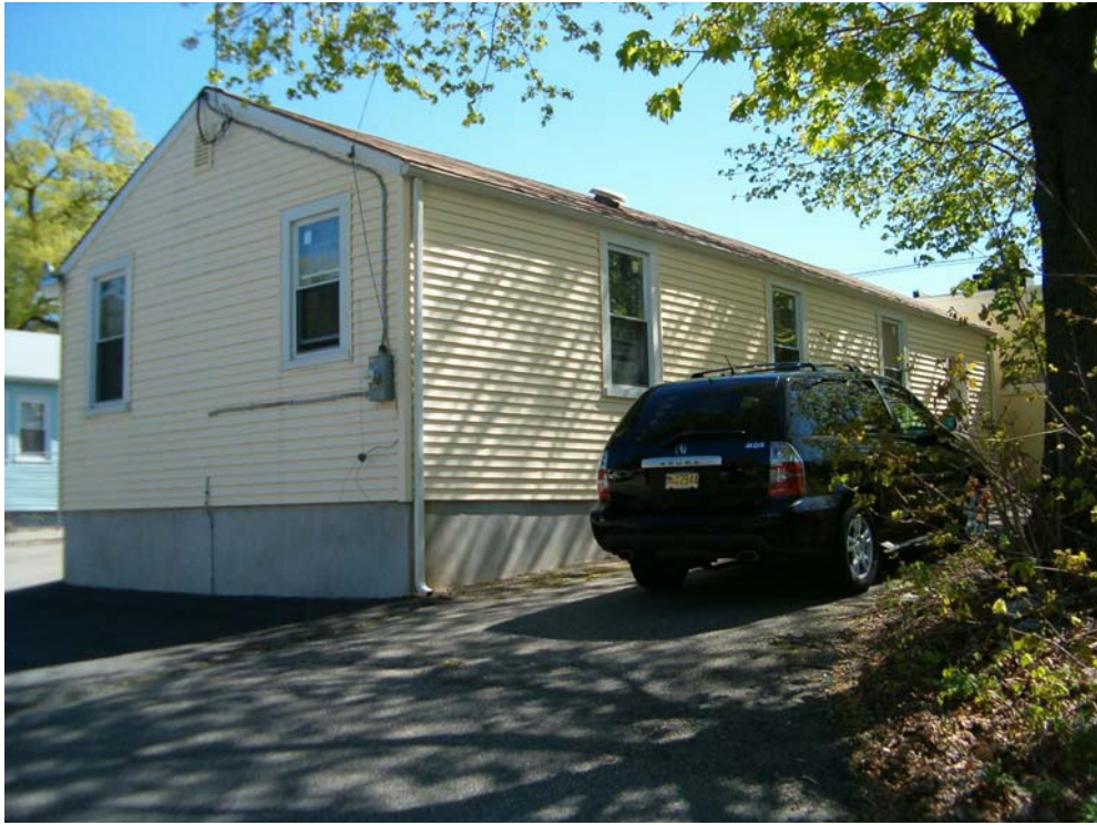
Building formerly occupied by Adrow Chemical Company.
