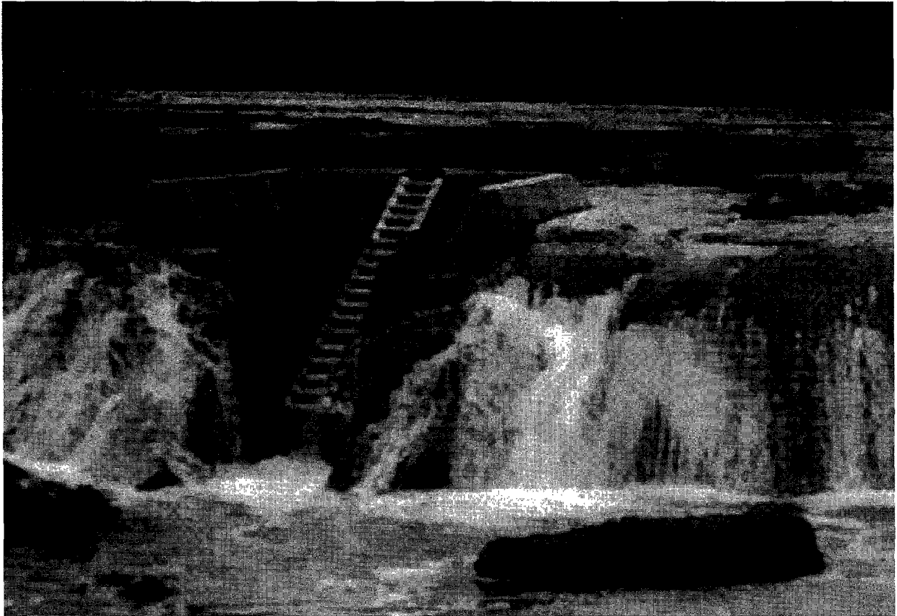
Keku Creek Fish ladder
