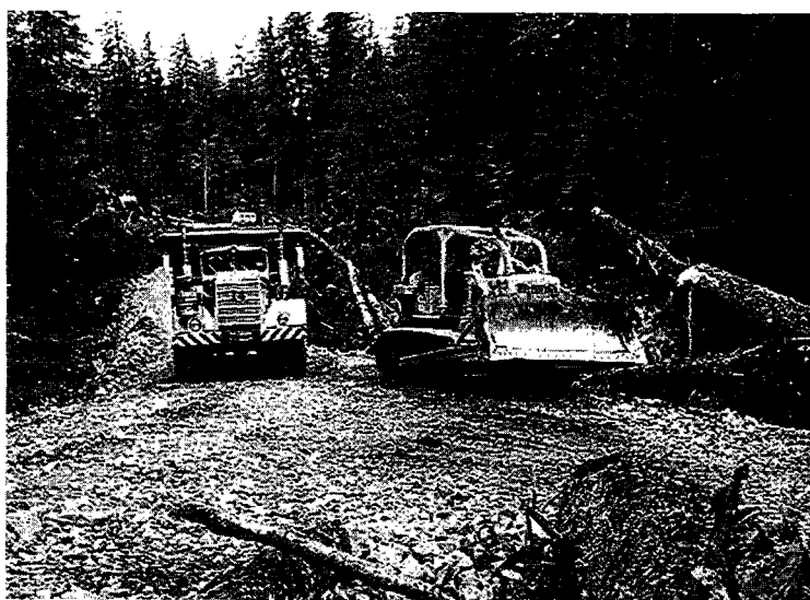
Heavy equipment building a new logging road
