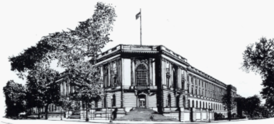
EXTERIOR OF THE CANNON HOUSE OFFICE BUILDING
