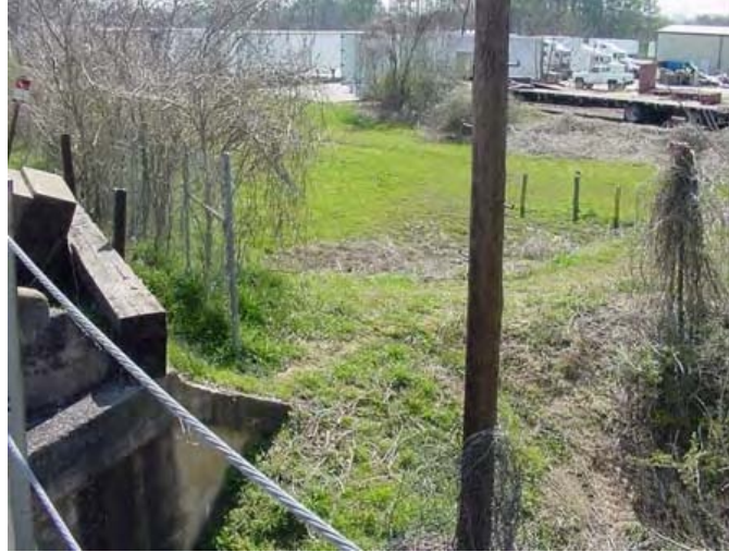
Gap along the northwest fence line ending at the levee adjacent to Cedar Creek west of the property. Entrance to property may be gained from the railroad tracks running along the northern property boundary. A groundwater monitoring well can be seen in the upper right area of the photo.
