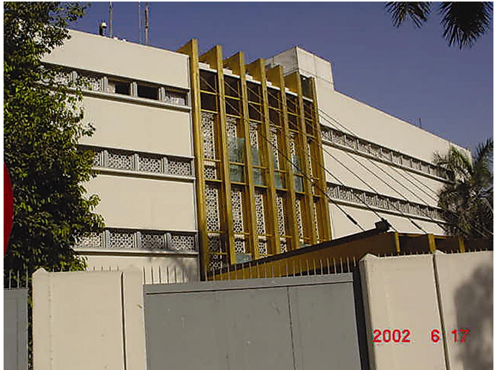
Figure 3: U.S. Consulate, Karachi, Pakistan, after Car Bomb Attack of June 14, 2002, Showing Little Damage to the Building
