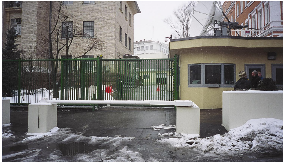
Figure 10: Newly Upgraded Compound Access Control Booth
