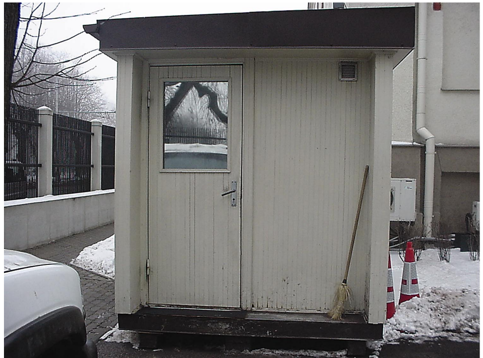
Figure 9: Inadequate Compound Access Control Booth
