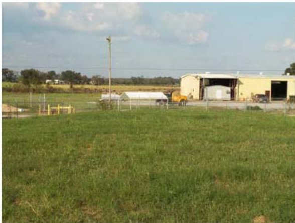
File Name: GSV_photo3.JPG Date/Time Taken: 01 Oct 2005 1636 Description: Eastern portion of cap, with equipment storage/maintenance facility in background, view to north. N29°57'28.1"; W92°11'11.4"
