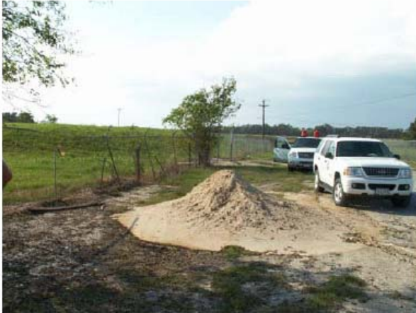
File Name: GSV_photo1.JPG Date/Time Taken: 01 Oct 2005 1625 Description: Fence line of site intact and not compromised by storm, view to west. N29°57'29.9"; W92°11'11.3"
