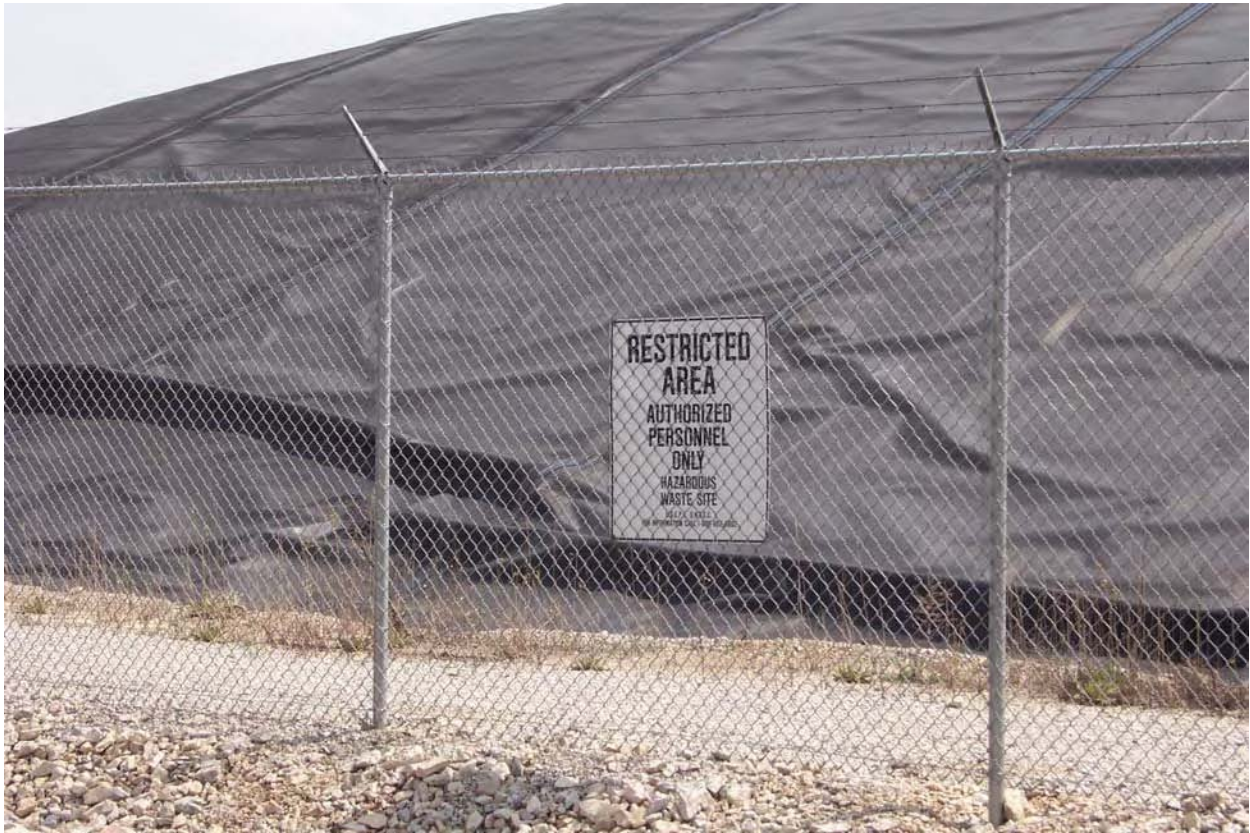
Figure 6. Slag pile covered with permanent 60-millimeter liner
