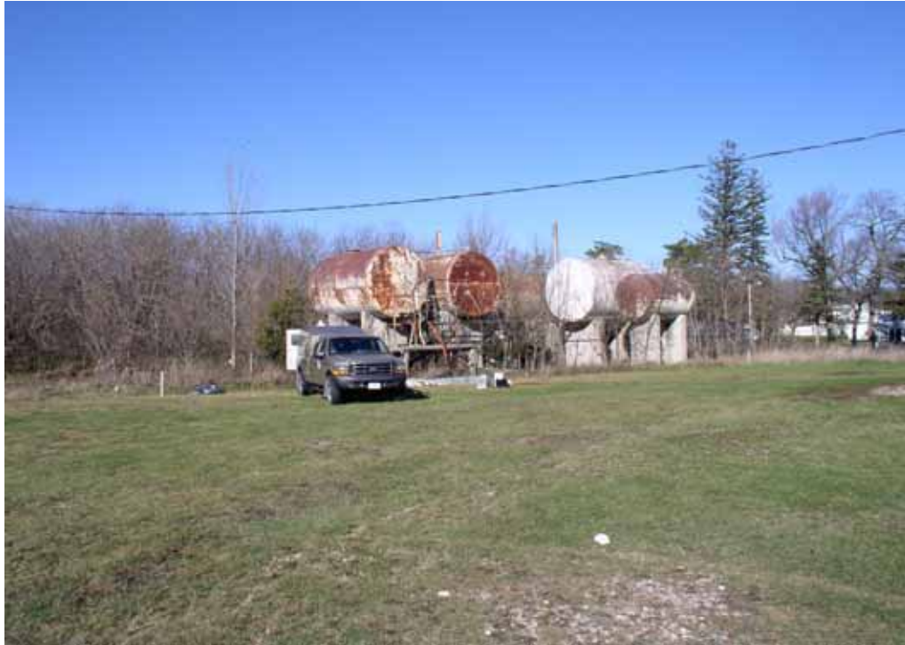
Photo 1 – View of Former AST Bulk Plant from the Southwest
