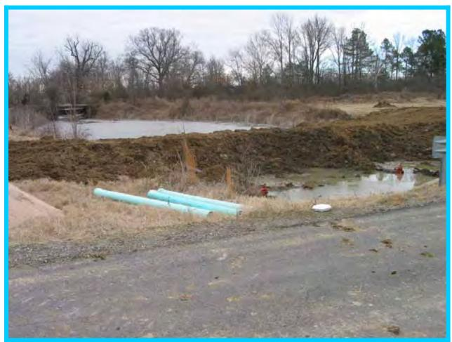
Figure 3. Photo of earthen dam on Railroad Creek to contain water used by fire department to fight the fire at Detco Industries.
