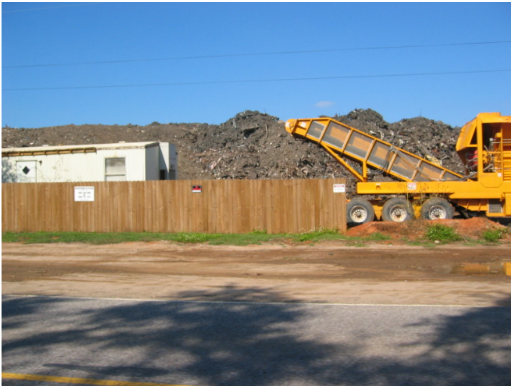
Photo 4: East of photo 3, (same trailer in both photos), before covering.
