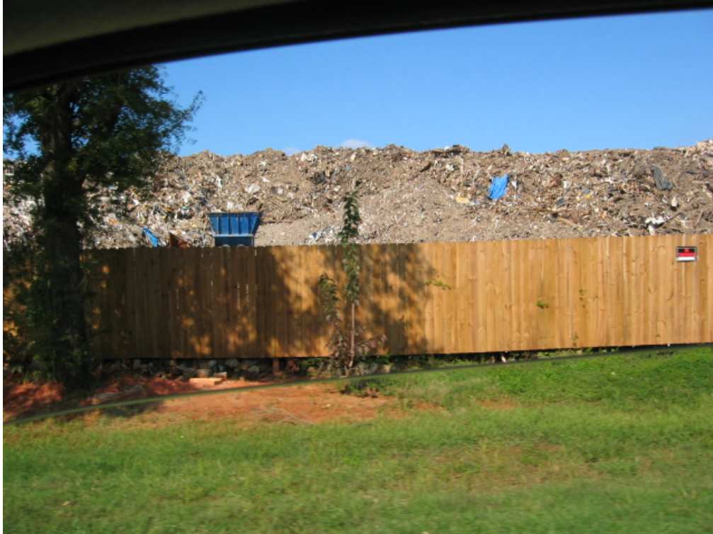
Photo 5: View of the Saufley Landfill from Saufley Field Road, southeast of the site, before covering.
