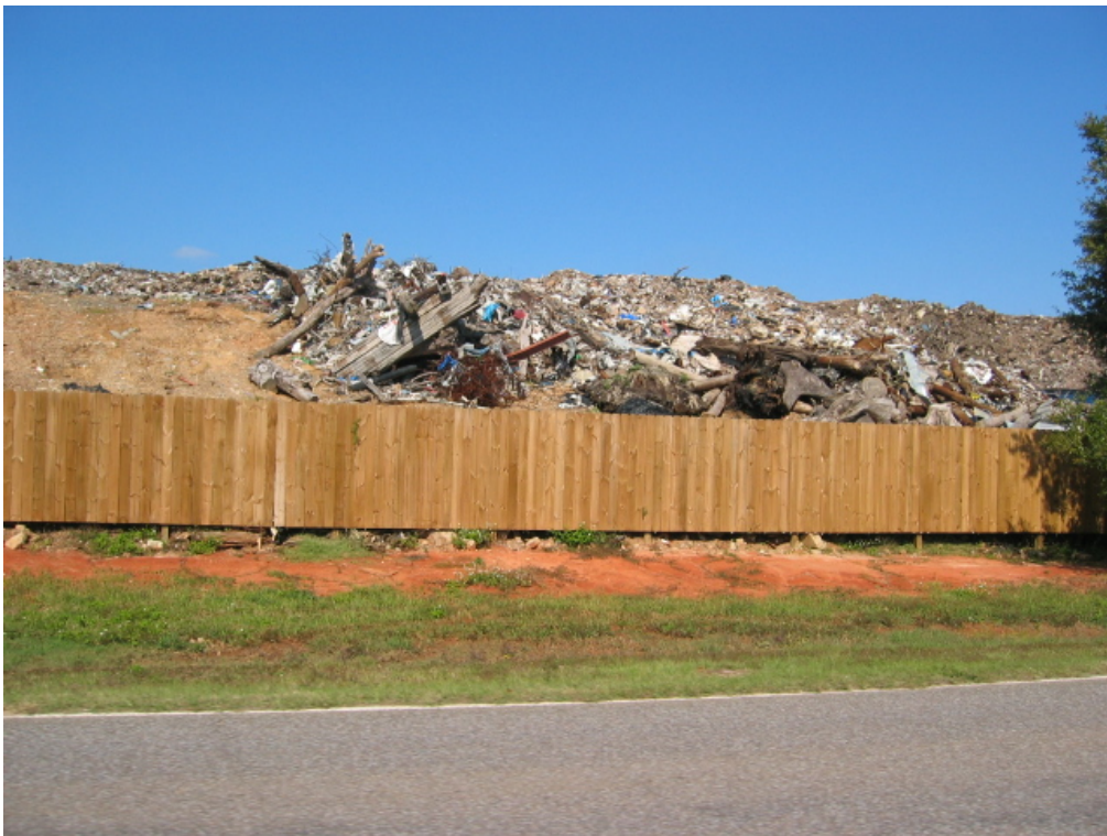
Photo 2: Close-up of Saufley Landfill from Saufley Field Road, south of the site, before covering.
