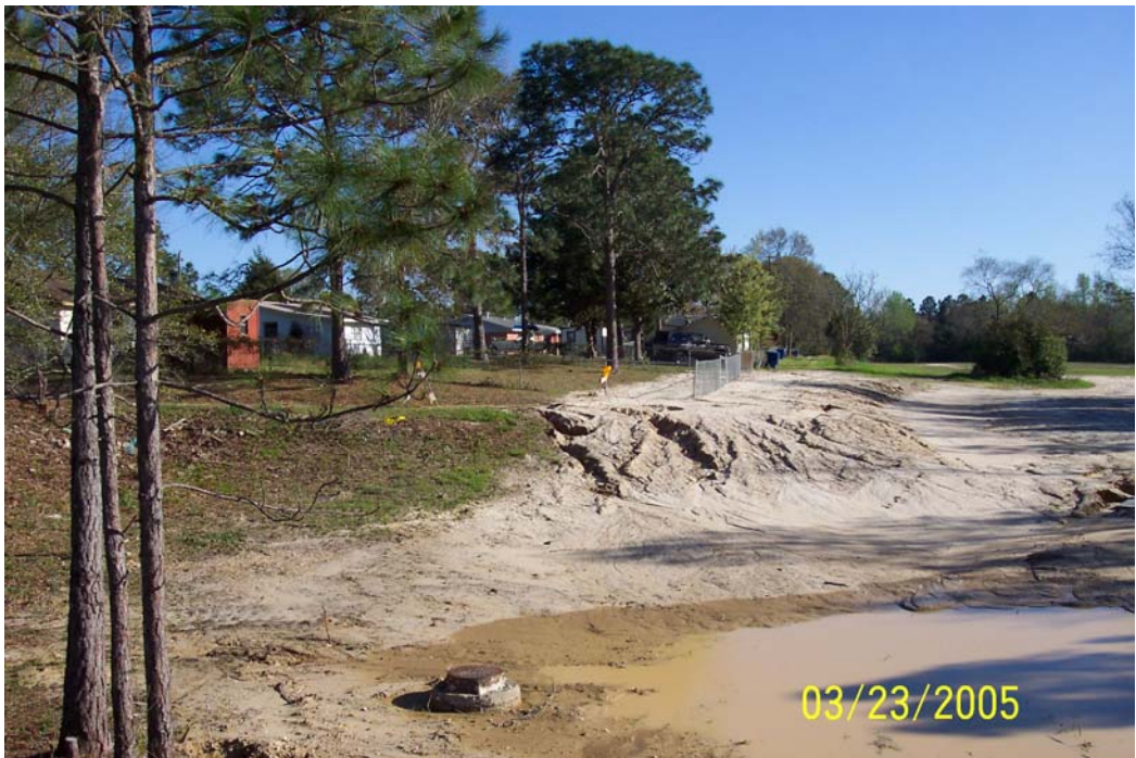
Photo 16: View of land subsidence from Seventh Street looking south.
