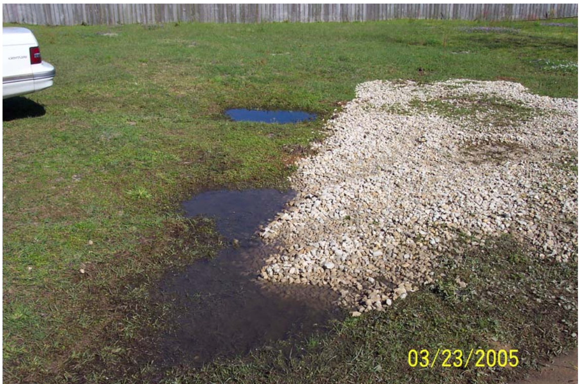
Photo 8: Holes developed near Flight Avenue in March 2005.
