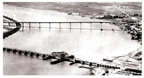
Victory Bridge, in foreground, is a swing bridge, pivoting on a center pier to allow boat traffic to pass through two channels. Opening the bridge in the summer resulted in huge traffic backups. Edison Bridge, west of the Victory, was built high enough to allow all vessels to pass under. Source: NJDOT
