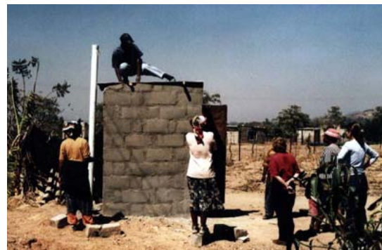
Allison (far right) working with villagers to maintain sanitation facilities.
