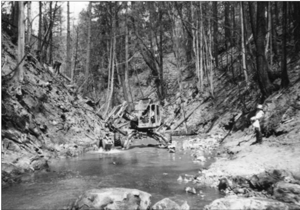
Figure 2. A track hoe "Spyder" used to agitate the stream bed and release trapped fuel.
