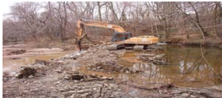
Dam Removal on Ridley Creek
