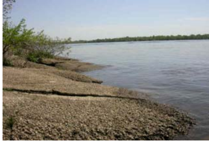
Poured Asphalt at Philly Coke Site
