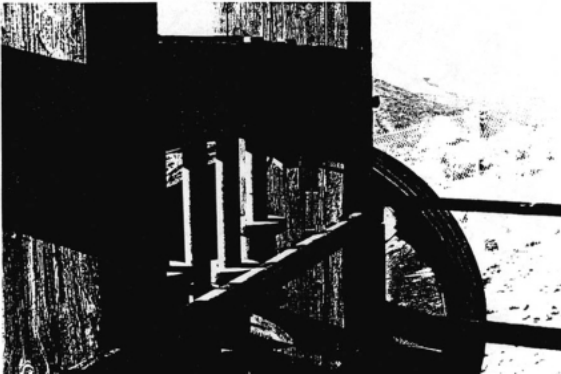
Fig. 7. Small entry to the ore bin on north side of Lost Horse Gold Mill. PSTU engineer entering the space below the ore chutes where core components were placed.
