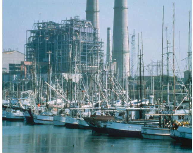
Figure HDD-1 – Moss Landing Harbor
