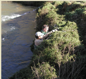
Service biologists perform stream restoration work (cedar revegetation) in Brushy Creek using bio-engineering methods. Brushy Creek is a tributary of Buck Creek which is home to four listed mussels. This was a cooperative project with NRCS. USFWS photo.
