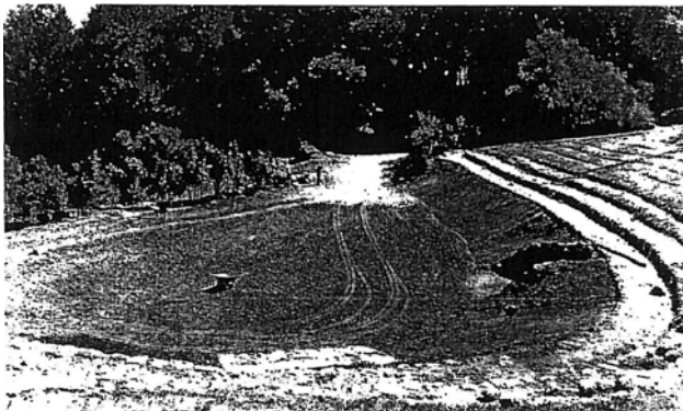
View to south. A screen of chicaquin oaks was planted as a backdrop to the stage. The sloped embankment separating the stage and auditorium was sufficiently high to accommodate the stone prompter's box seen in the mid right portion of the photo. The finish grading of the stage is completed by hand and readied for a wild flower sod that was collected from a nearby grassland. (Courtesy of the National Archives)
