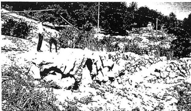
View looking northwest. Stone retaining walls were constructed to support the approximately twelve foot of fill in the ravine that once crossed the stage. These walls also provided a system of ramps that allowed actors to move from stage left to stage right without being seen by spectators. (Courtesy of the Marin Historical Society)
