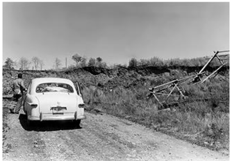
FIGURE 3: Photograph of a splay of the Red Canyon fault scarp created a 10-foot wall across the road. Photo by Carl Hayden, Salt Lake Tribune. (University of Utah, 2007)
