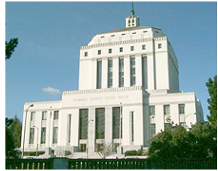
The Alameda County Courthouse is one of 50 county facilities receiving a lighting upgrade. The project is expected to save the county hundreds of thousands of dollars annually in electricity consumption. (Photo courtesy of Alameda County)
