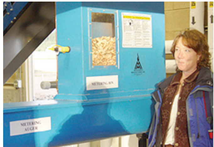
Nan Christianson, state and private forester in the U.S. Forest Service Northern Region, watches the metering bin feed the new biomass boiler at the Darby, Mont., schools. (Photo by Montana Division of Natural Resource Conservation)
