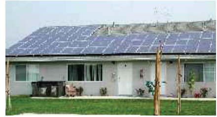
PV panels on the roof of the Autumn Ridge affordable apartment complex reduces resident's electric bills. (Photo by Riverside Housing Development Corporation)
