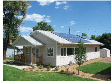
Habitat for Humanity partnered with National Renewable Energy Laboratory to build its first true net-zero-energy home in Wheatridge, Colo. (Photo by Paul Norton)
