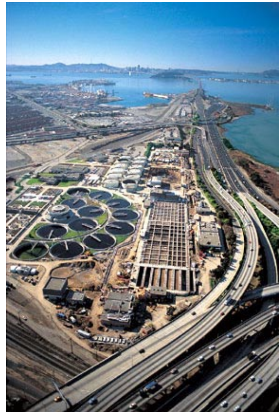
EBMUD's main water treatment facility, produces 75 percent of its own electricity from biogas captured during the treatment process. (Photo by East Bay Municipal Utility District)
