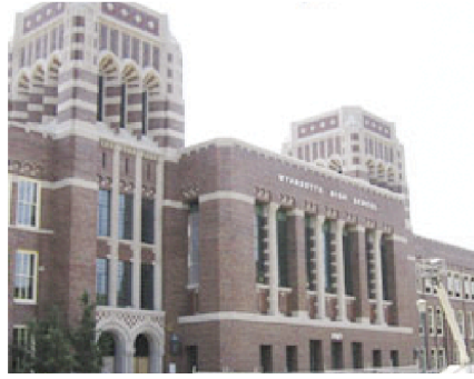
Converting facilities like Wyandotte High school from gas to electric heat helped Kansas City, Kan., Public School District to save thousands of dollars in annual operating costs. (Photo courtesy of KCKPS.)
