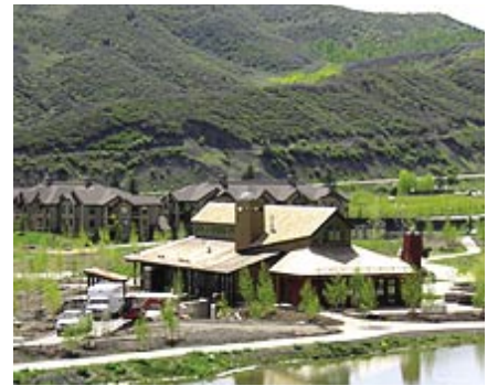
The Snowmass Golf Clubhouse in Aspen, Colo., was built with the latest in green construction technology. Owner Aspen Skiing Company has applied for a LEED gold certification. (Photo courtesy of Aspen Skiing Company)
