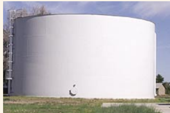
The blended water in this 750,000-gal. water tank supplies Julesburg residents with clean, safe water that meets the state's standards for nitrogen concentration. (Photo courtesy of Julesburg Utilities)
