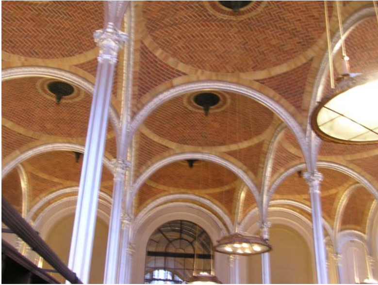
Figure 56: The view of rib and dome construction.
