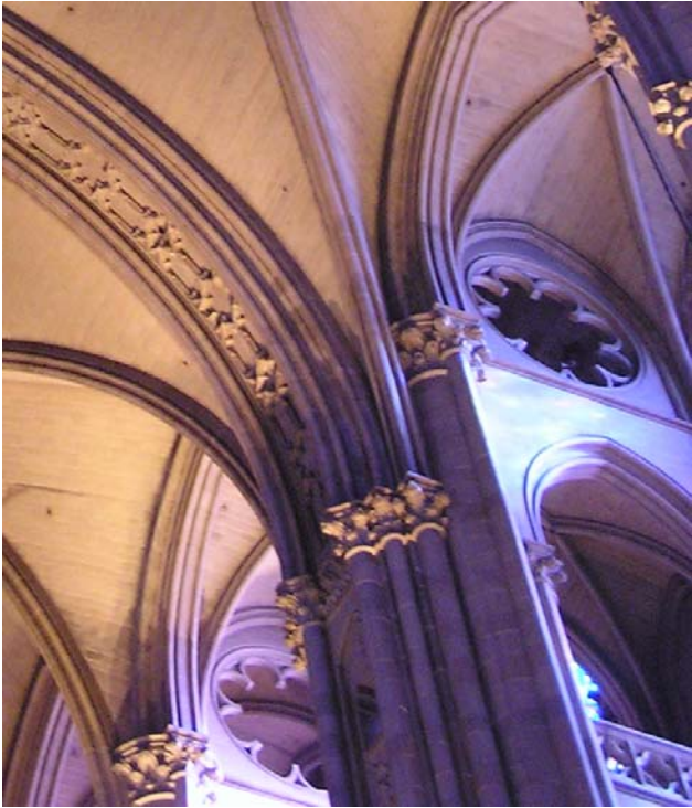
Figure 28: Vault Rib Intersection at Springing
