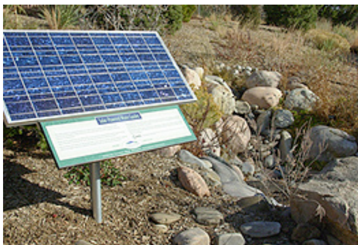
Solar panels power the pump that runs the waterfall in the xeriscape garden at the Colorado Springs Utilities Conservation and Environmental Center.
