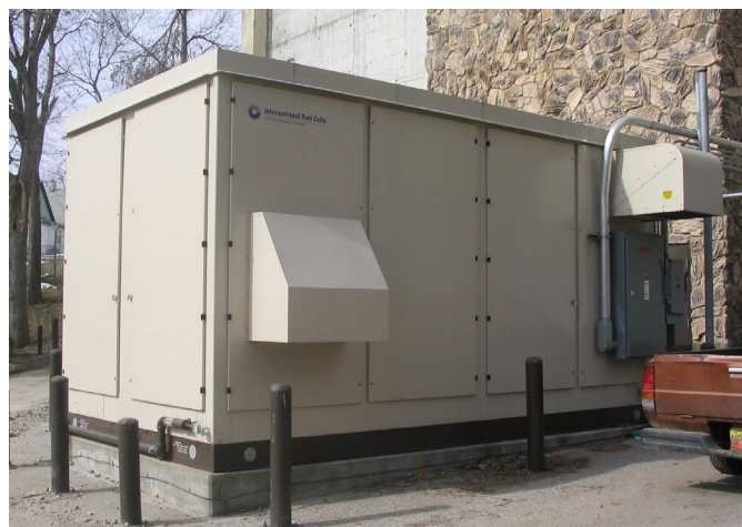
The 200-kw fuel cell OPPD installed at Omaha's Henry Doorly Zoo quietly powers the Lied Jungle indoor rain forest and heats water with captured waste heat. (Photo by the Henry Doorly Zoo)
