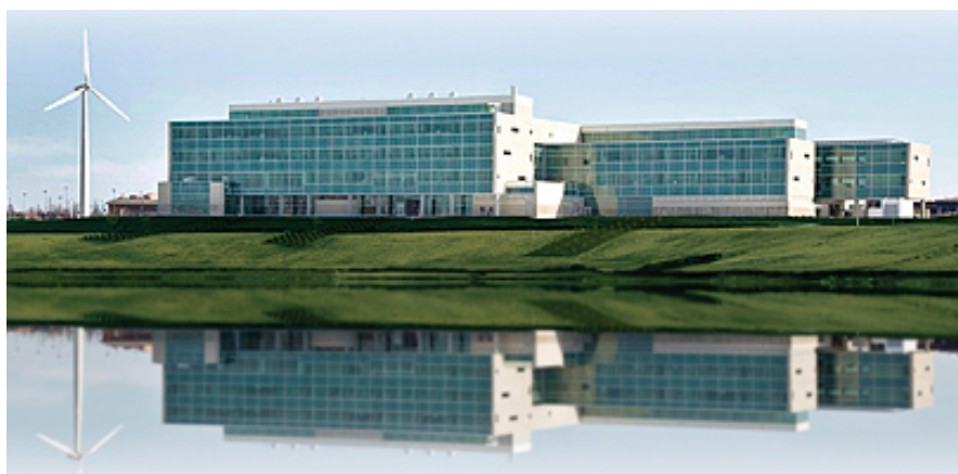
Energy efficiency can be beautiful, as Great River Energy's new headquarters in Maple Grove, Minn., proves. Project leaders are submitting the 166,000-sq. ft. building for LEED platinum certification. (Photo by Great River Energy)
