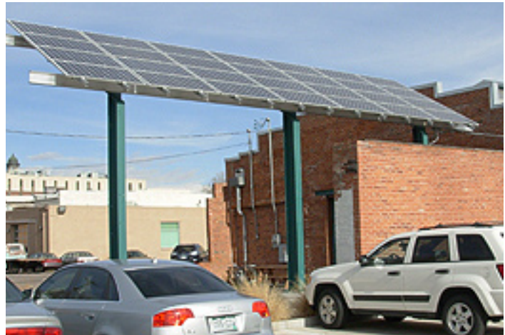
The bike shop parking lot was the second choice for siting the solar array, but made little difference in system performance. (Photo by Gary Hoffmann)
