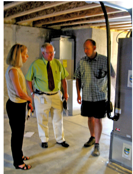
Jammie Sabin (left) of Aspen Homes discusses the advantages of the all-weather, air-source heat pump with Energy Services Representative Linda Swails and Mike McCoy of Tri-State G&T.
