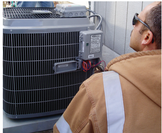
Warren Neal of Loveland Water and Power installs a cycling device on a customer's air conditioner. Customers are volunteering for the cycling program to help the utility manage its summer peak. (Photo by Loveland Water and Power)
