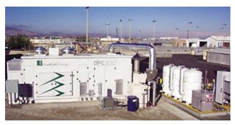
This fuel cell and waste heat recovery unit provides 36 percent of the power needs of the Palmdale, Calif., water reclamation plant. (Photo by Los Angeles County Sanitation Districts)
