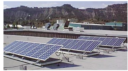
The Jicarilla Apache Nation of New Mexico, one of Western's new customers, installed a 2.4-kw photovoltaic system on the Dulce High School, and monitored its performance for three years. (Photo by DOE Office of Energy Efficiency and Renewable Energy)
