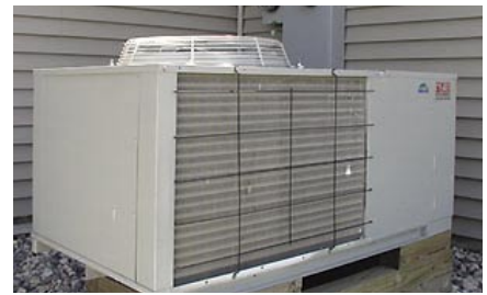
Cass County Electric Cooperative Marketing Manager Marshal Albright of installed this CCHP at his Fargo, N.D. home. (Photo by Cass County Electric Cooperative)
