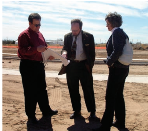
Architects Dean Cruse (Durham/Kilmer), James Crockett (NPS), and Nancy Cocroft (NPS) inspect the NCKRI building site.
