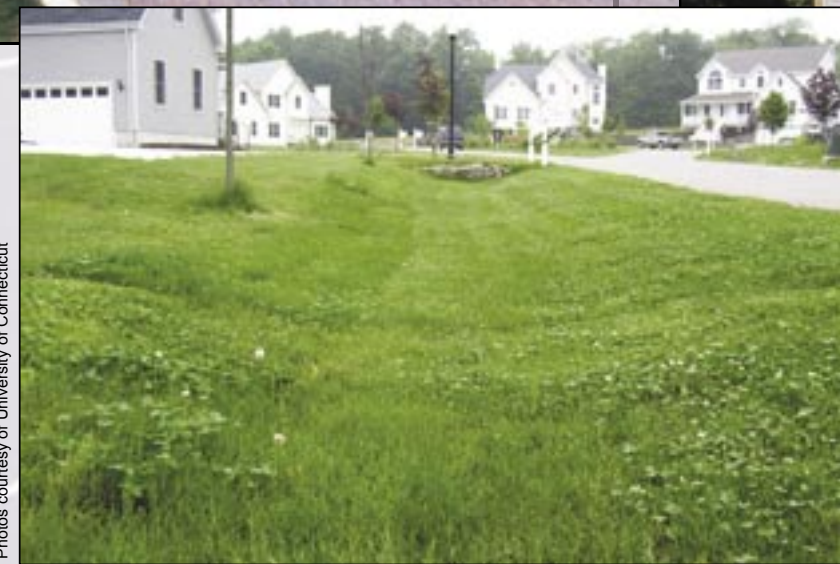
The experimental Jordan Cove project features (clockwise from top) a narrow road made of permeable paving blocks, rain gardens that absorb roof runoff, and grass swales.
